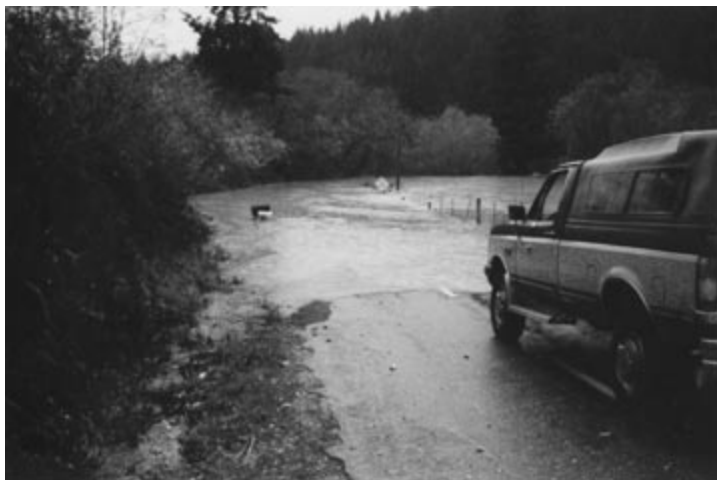
An inundated bridge on Elk River Road is normally 20 feet above stream.
