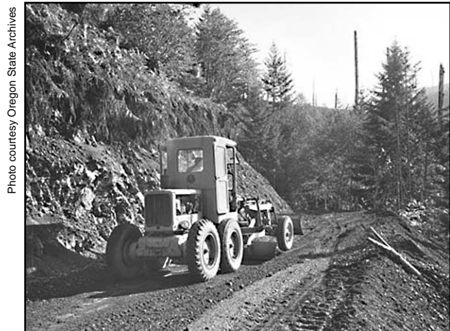
Roadbuilding in the Tillamook Burn, Oregon, 1953
